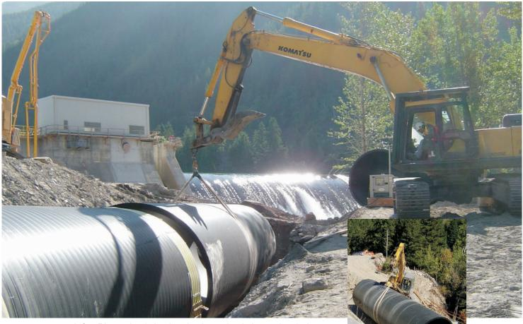
Infra Pipe raised the bar in the polyethylene pipe industry when it produced Weholite pipe for the Aberfeldie Runof-River Hydro redevelopment project.
